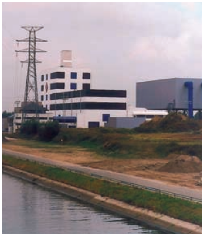
Combined heat and power plant (360MW) for Electrabel (Ghent - Belgium)
