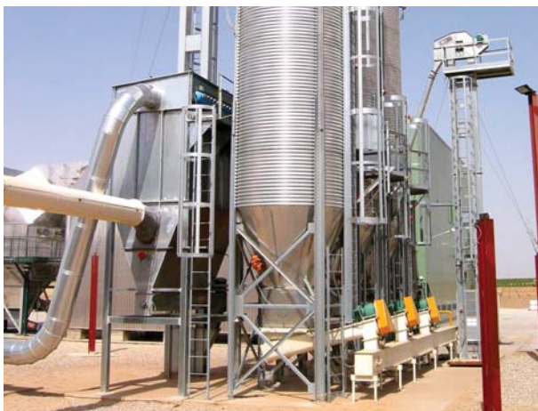
The entire wood waste energy conversion process at the Villacañas biomass factory is equipped with LS motors, geared motors and an alternator, all certified to operate in explosive atmospheres (ATEX dust).
