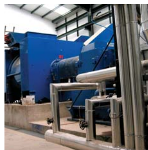
The entire wood waste energy conversion process at the Villacañas biomass factory is equipped with LS motors, geared motors and an alternator, all certified to operate in explosive atmospheres (ATEX dust).
