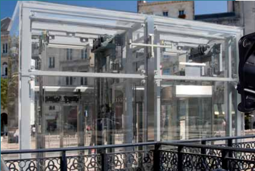
Lift zonder machinekamer (Bordeaux) Gamma XA gearless motor XAP2M
