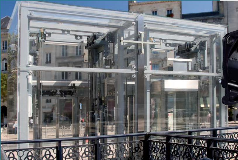
Machine roomless lift (Bordeaux) XA range Gearless motor XAP2M
