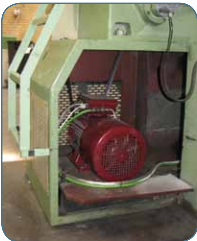
... was replaced by an energy-efficient LSRPM motor.
