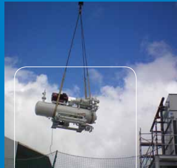
A compressor with its Leroy-Somer electric motor is winched into place at the food production plant.
