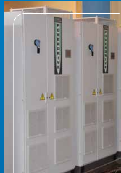
Leroy-Somer electric motor control panels in the electrical supply room at the factory.
