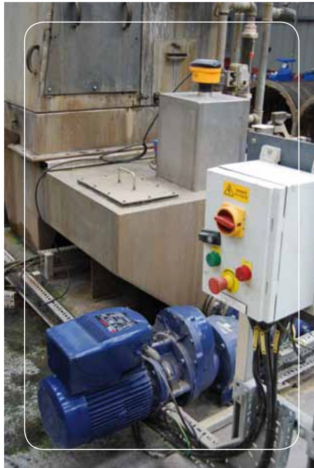
The new system with the Leroy-Somer Varmeca 30 inverter-based variable speed motor now operates without problems.
