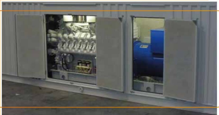
Backup diesel generator installed in a processing factory located at M'Boundi in the Republic of Congo.
