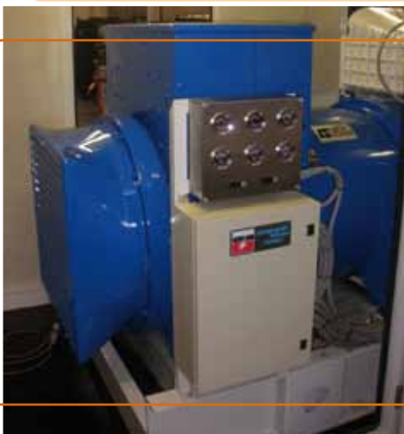
Alternator from the expanded low-voltage range LSA 53.1 M80/4P - 2300 kVA - 400 V
