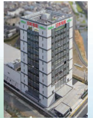
NIDEC CORPORATION HEAD OFFICE ANNEX GLOBAL LEARNING CENTER
